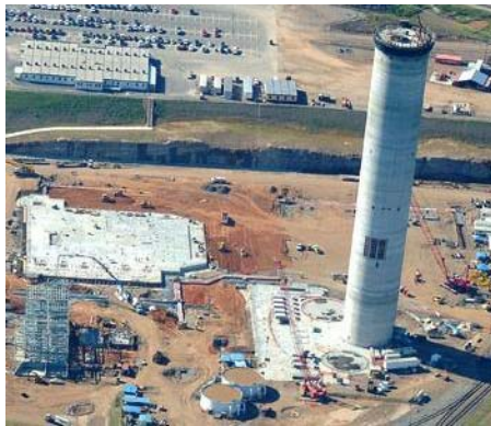
CLIFFSIDE PLANT CONSTRUCTION
